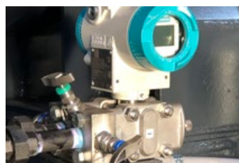
MODULATING MAKE UP CONTROL VALVE WITH DIFFERENTIAL PRESSURE TRANSMITTER
