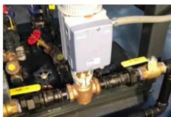
MODULATING MAKE UP CONTROL VALVE WITH DIFFERENTIAL PRESSURE TRANSMITTER
